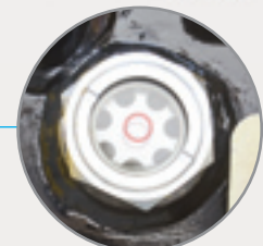
Hydraulic Oil Level Gauge
